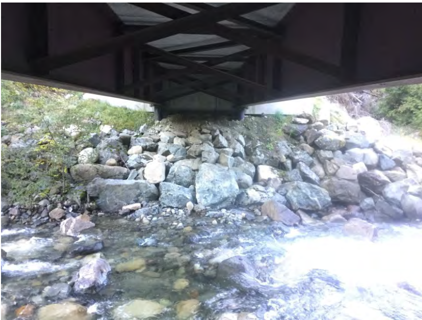
Left Bank Abutment when facing downstream
