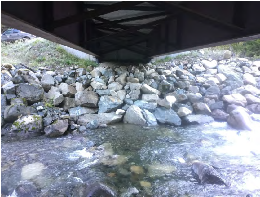
Right Bank Abutment when facing downstream
